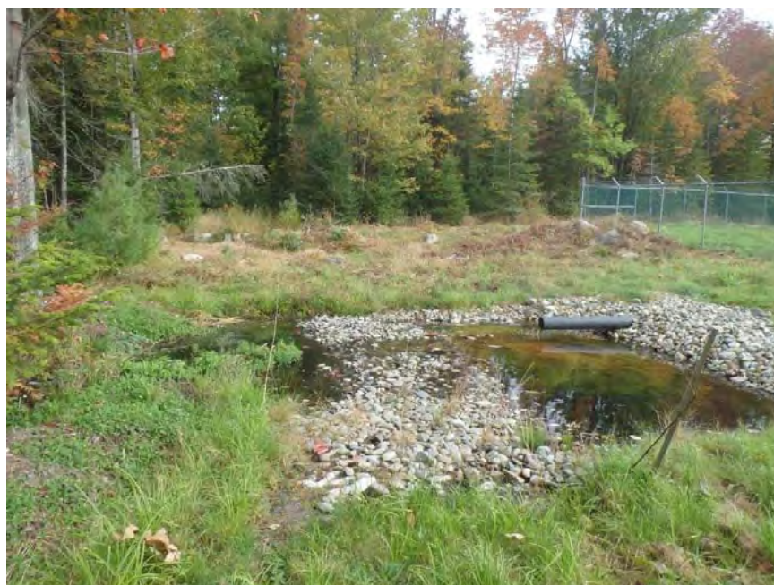
Photo 2. Stormwater pond outlet pipe draining into Wetland 01TTA. Stantec, September 25, 2014.
